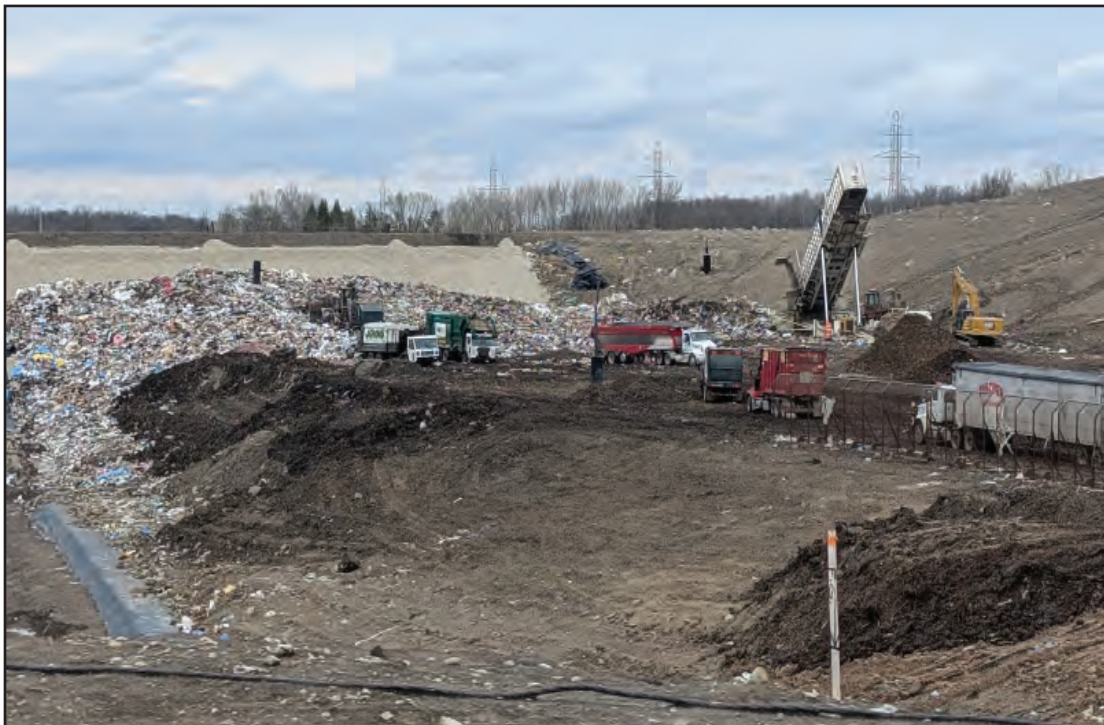
Working face viewed from West
