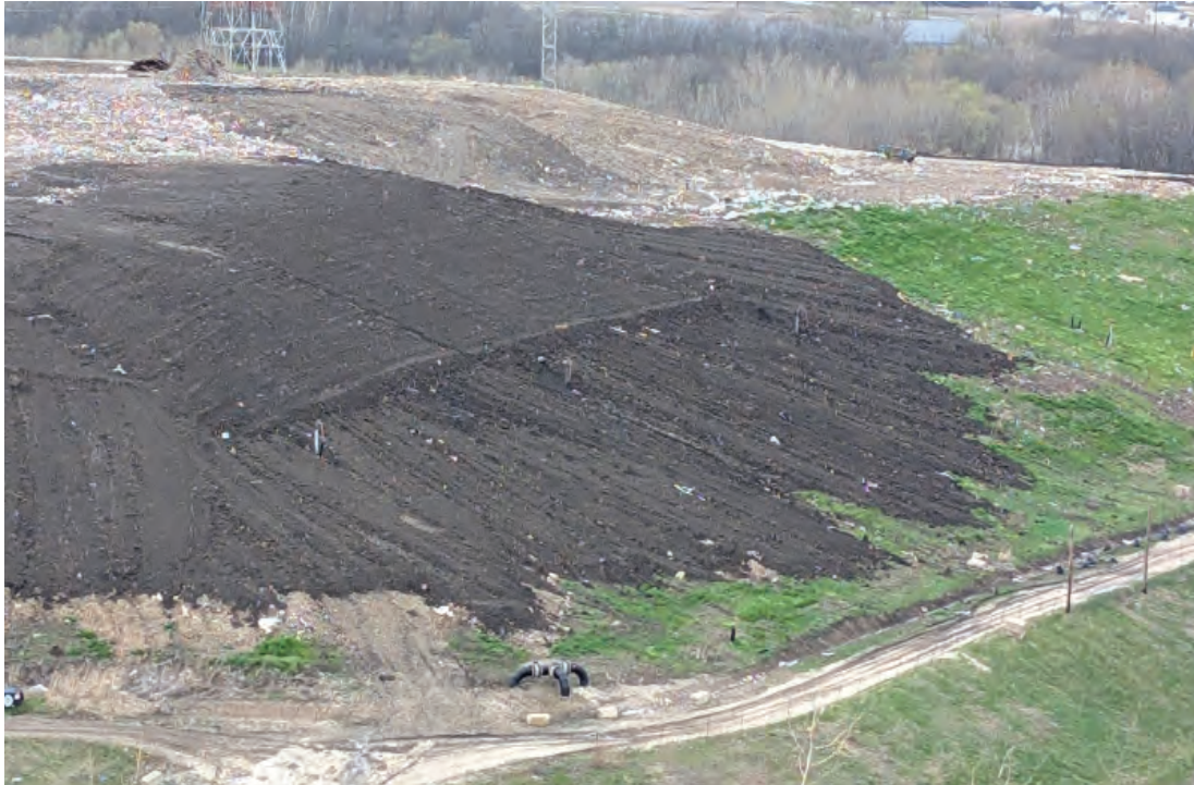
Top soil spread on East sope of Phase
