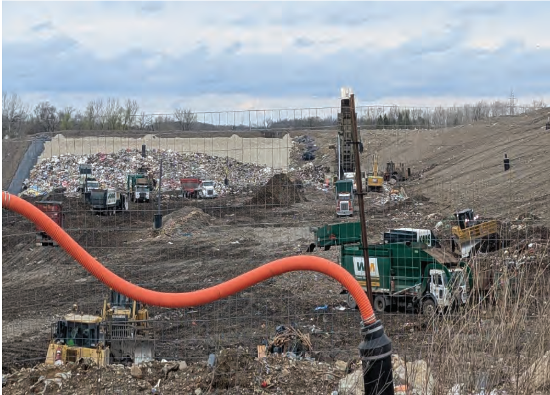
Trucks cleaning out against Phase 3, from Phase 4. Working face in North end of Phase 4
