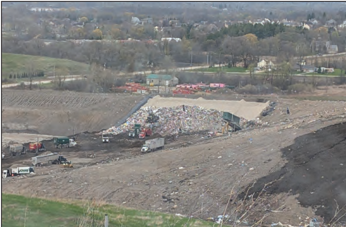
Working face at North end of Phase 4, starting new lift
