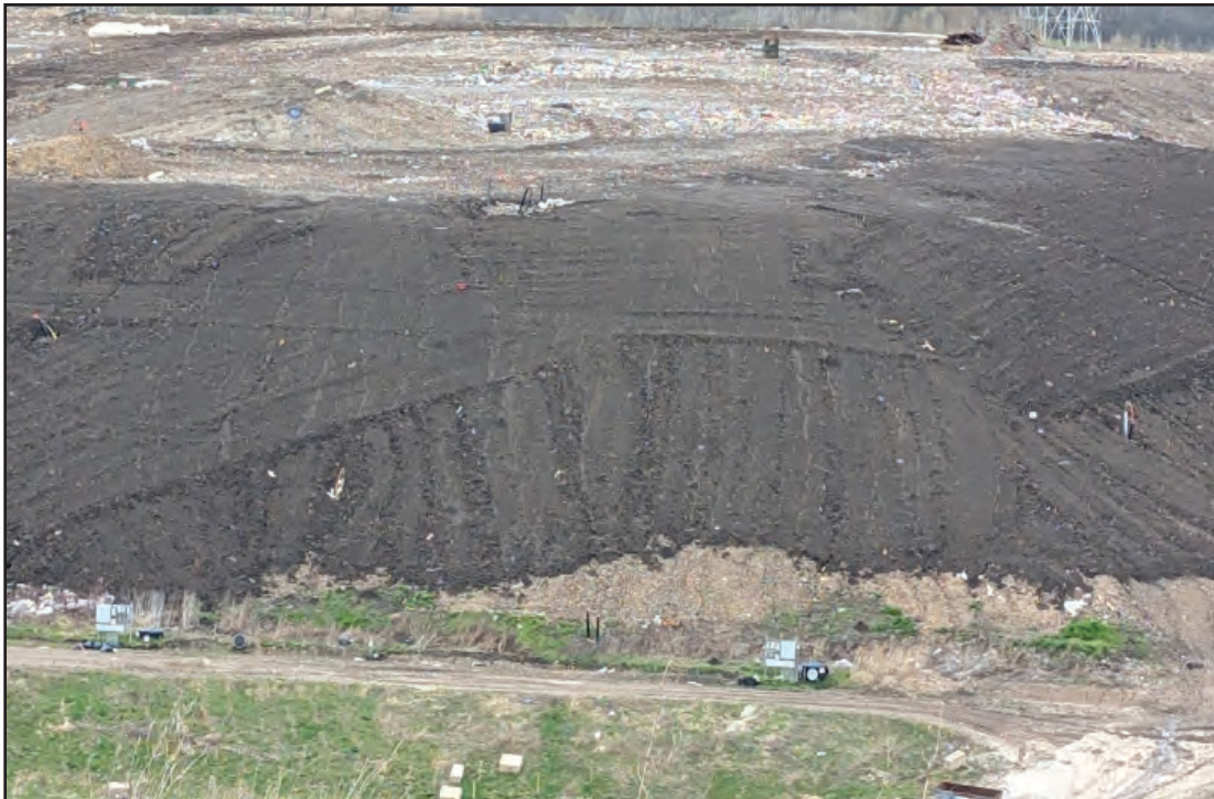
Top soil well spread over South slope and East slope of Phase 1
