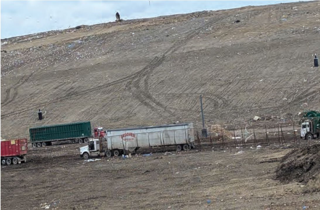
Long haul vehicles entering from Phase 3 West slope
